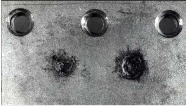
Figure 3-7. Spot Weld Corrosion
