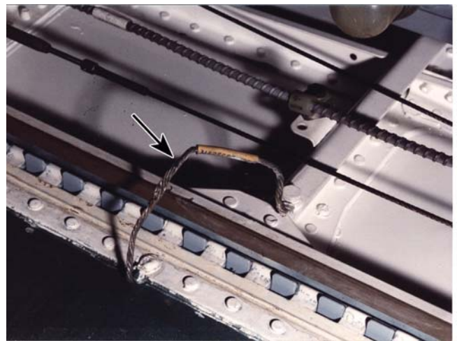
Figure 6-4. Bonding Cable From Airframe to Graphite/Epoxy Avionics Bay Door
